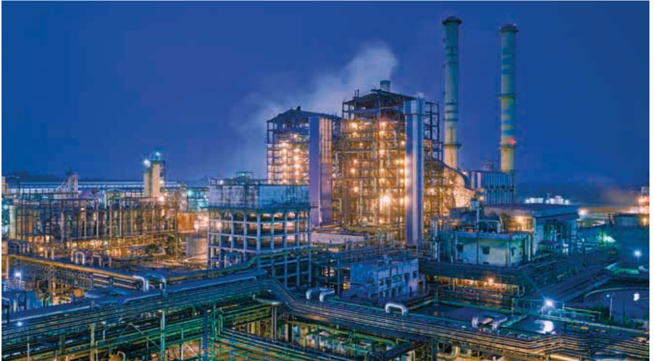
ITC's Paperboards Factory, Bhadrachalam
