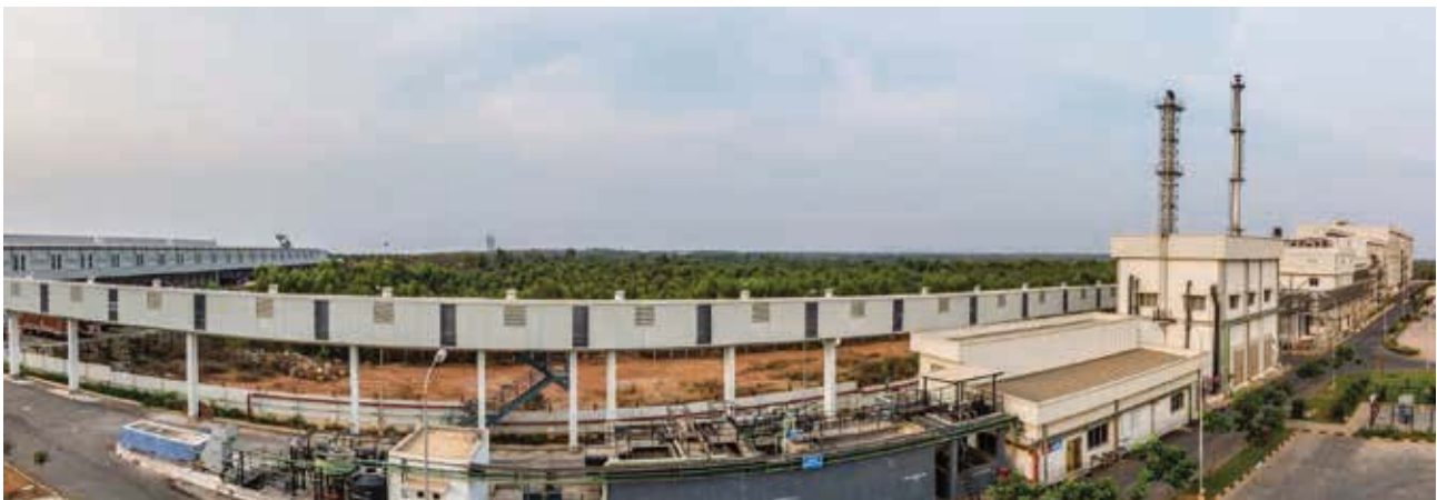
ITC's Integrated Consumer Goods Manufacturing Facility, Malur
