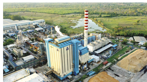
The High Pressure Recovery Boiler at Bhadrachalam significantly enhances the paper plant's energy efficiency and ITC's decarbonisation efforts
