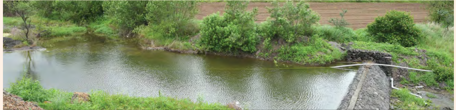
Check Dam in Maharashtra
