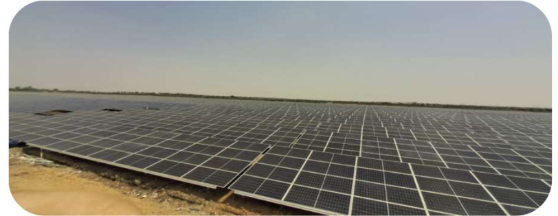
Solar Plant, Karnataka
